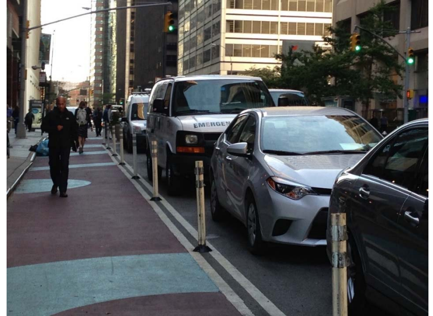
Separated Trail on Existing Asphalt
